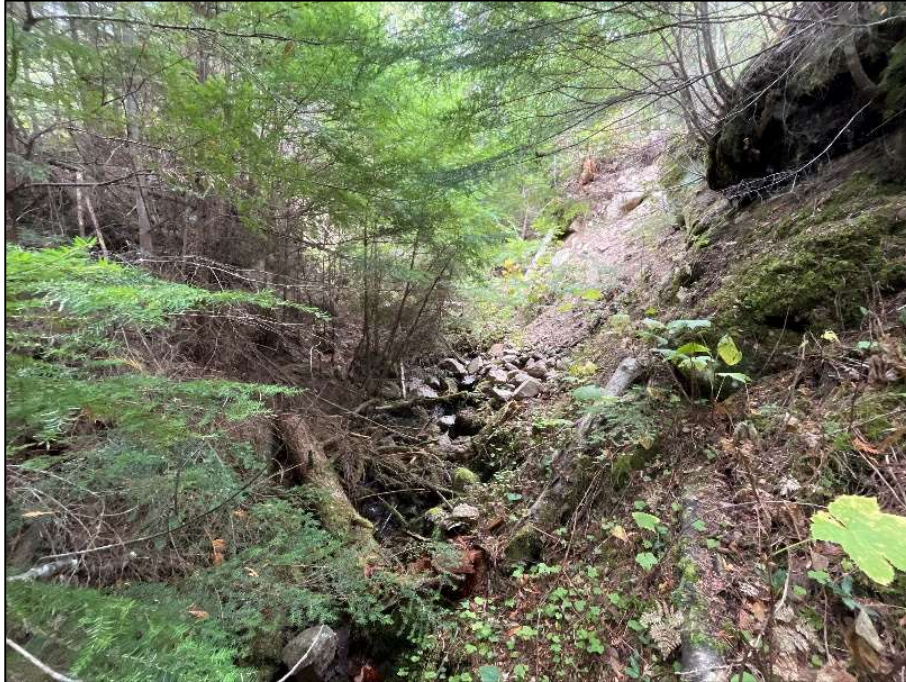
Photo 13: Cory Middle Creek along the fire guard (Field Observation Site K54). Note the trim line along the bank to the right, this is evidence of passage of a recent debris flow.
