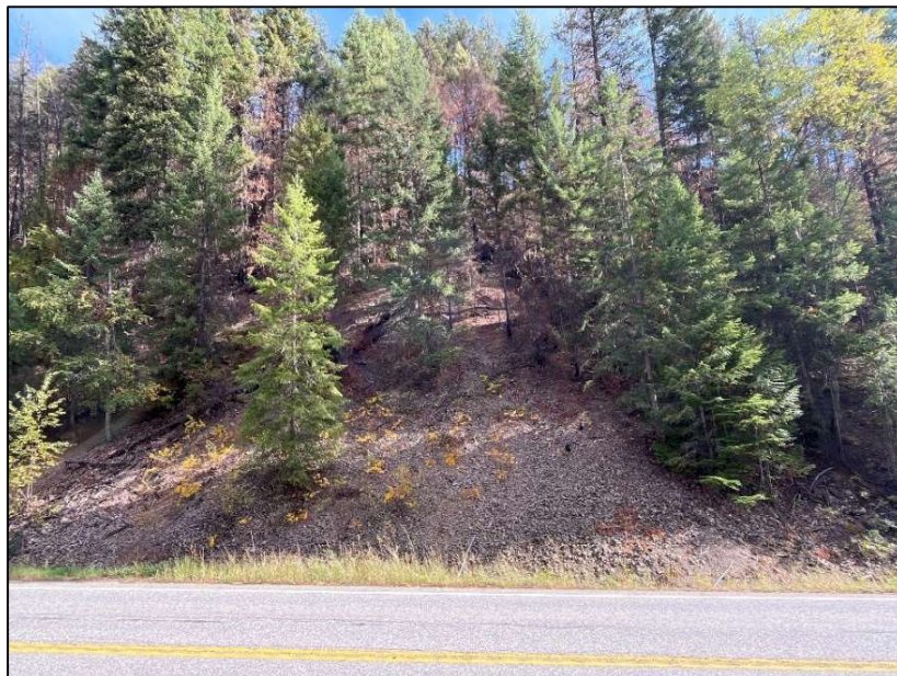
Photo 28: View of a moderately steep rubbly talus cone exposed above the Highway near the Slokan Lake View Point (Field Observation Site K29). Removal of the surface vegetation has decreased the stability of the slope and rock fragments are moving downslope into the ditch.
