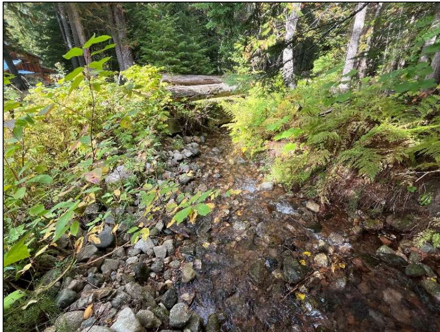
Photo 21: View downstream along Fingland Creek from the access road to 8473 RMR (Field Observation Site K4). The creek has a low gradient and is contained in a shallow swale. The residence, visible at upper left, is located 50 m from the creek on a flat bench and is potentially vulnerable to flooding or creek avulsion.
