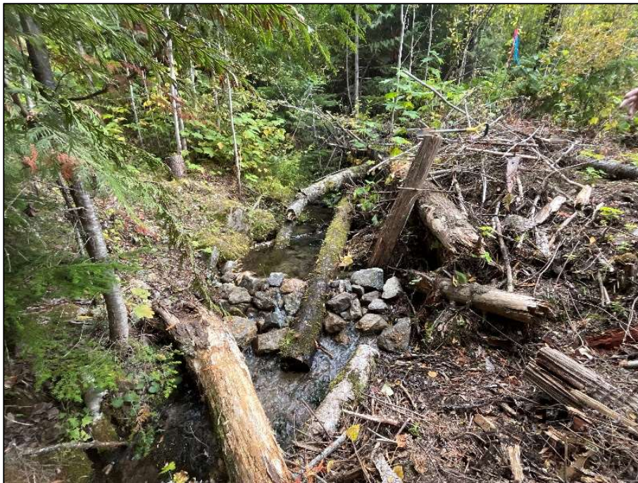
Photo 14: Cory North Creek along the fireguard (Field Observation Site K55).
